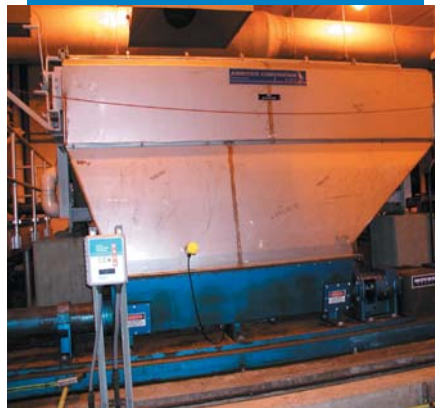
Pump, base, drive, hoppers, controls ... Moyno has extensive experience in building complete pumping units like the one pictured here handling dewatered sludge.
