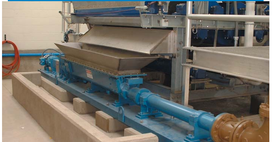
The Moyno 2000 G3 filter cake pump has proven to outperform and outlast all other pumping alternatives in dewatered sludge cake applications.
